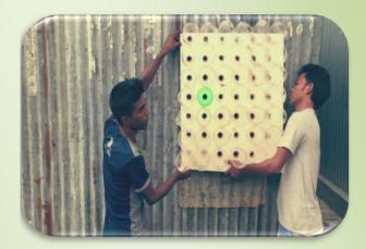
Do you have a few plastic bottles lying around? Then you can make an air conditioner - really. Eco-Cooler is a low-cost cooling system designed for developing regions. It's constructed from halved plastic bottles inserted into a grid-like board, which is then installed in a hut like a window pane.
